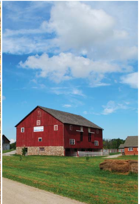
Spruce Lane Farmhouse
